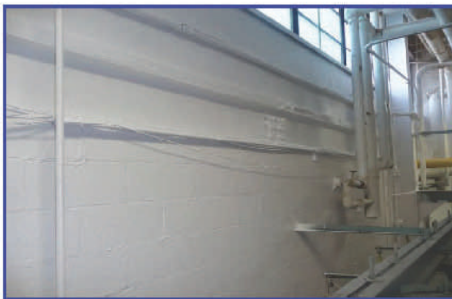
This wall, inside a food processing plant, is coated in Jaxsan 602 and Jaxsan AG-102.
